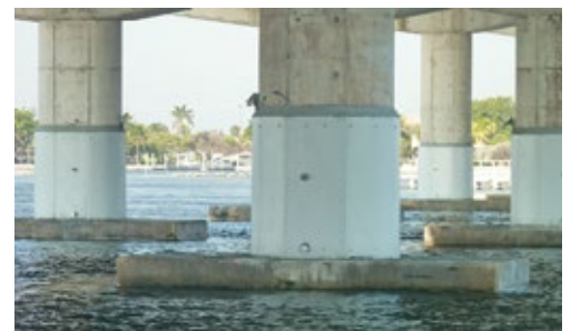
Galvanode DAS Jackets Installed
