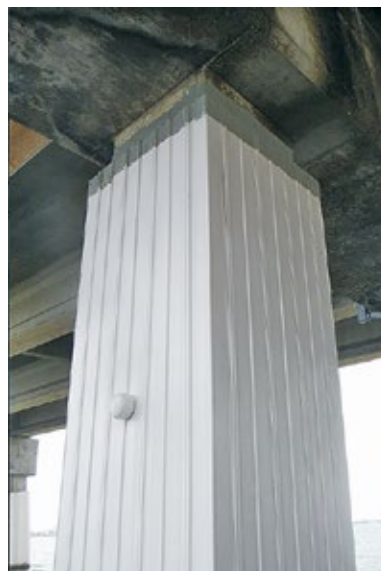
Galvashield Tidal Plus Jacket with Modular PVC Stay-in-Place Formwork
