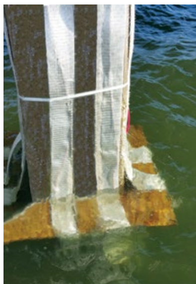
Galvashield Tidal Plus Jacket with Wicking Fabric Anodes (prior to jacking)
