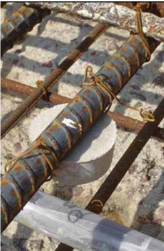
Fig. 3: Sacrificial anode installed within concrete repair area
