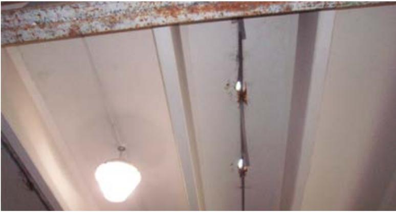
Fig. 4: Tee flange joint failure
