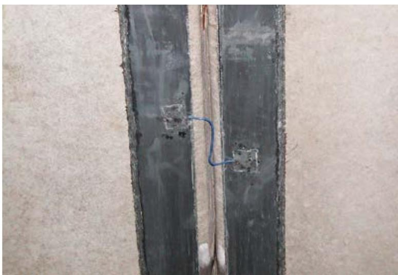
Fig. 12: Zinc sheet protecting damaged and undamaged flange connections
