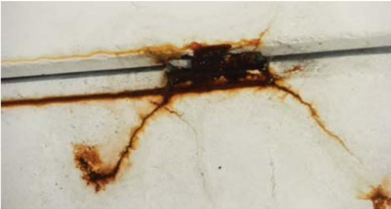
Fig. 5: Corrosion of tee flange connector
