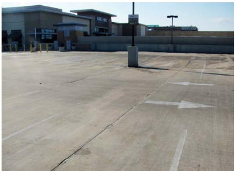
Fig. 3: Precast double-tee deck
