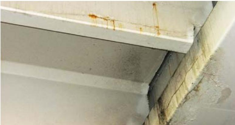
Fig. 6: Double-tee stems and inverted T-beam haunch
