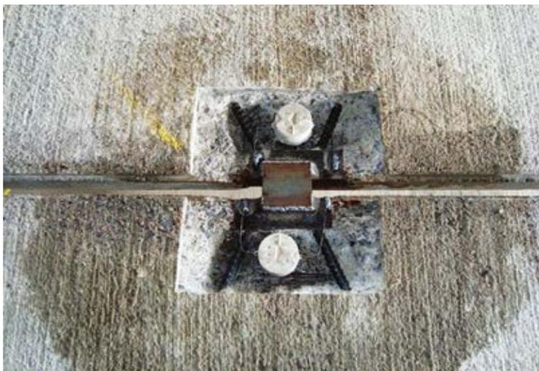
Fig. 11: Discrete galvanic Type 1 anode protecting flange connector
