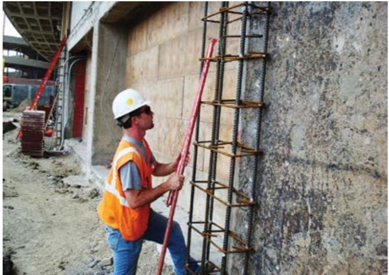
Fig. 15: Galvanic strip anode installation within reinforcing cage
