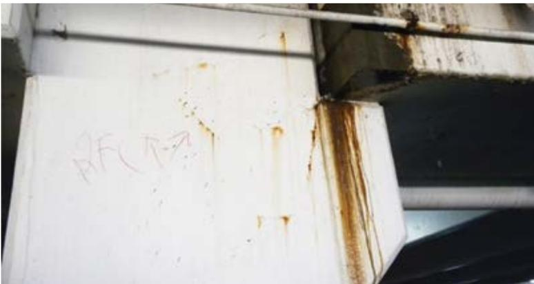
Fig. 7: Inverted T-beam and column corbel
