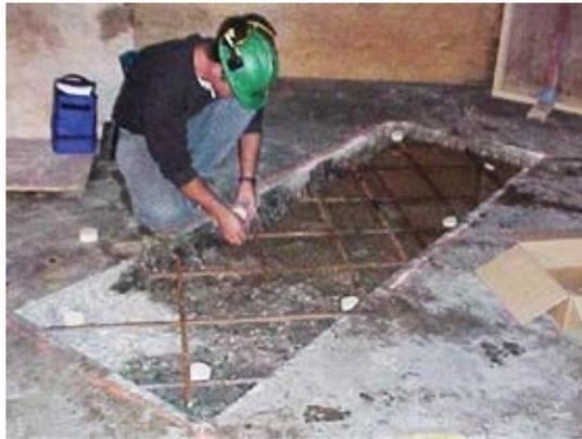
Fig. 8: Discrete galvanic Type 1 anode installation
