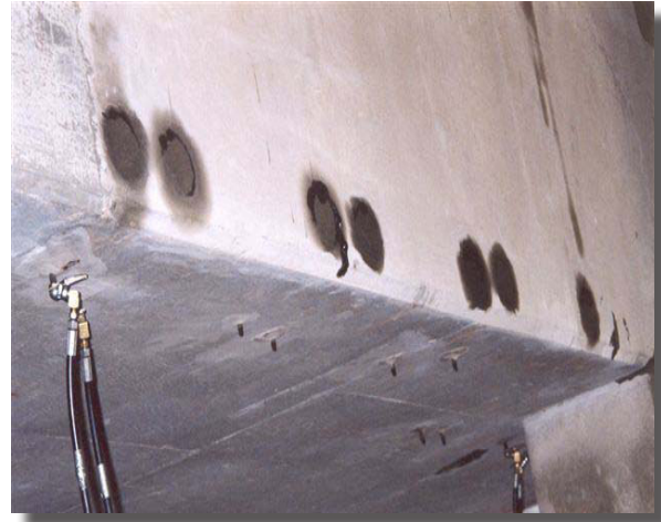
Post-Tech PT Grease Injection
