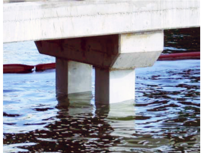
Galvashield Tidal Jacket provides protection to pile section in the tidal zone
