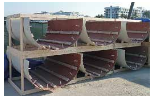
Galvashield DAS Jackets Prior to Installation
