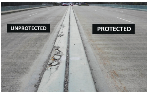
Steel-reinforced Concrete Roadway
