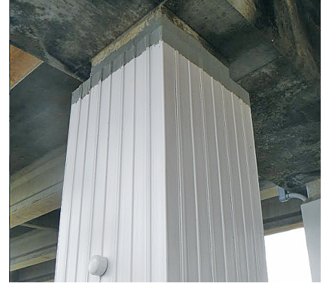
Galvashield Tidal Plus Jacket provides protection to pile sections in the tidal zone and above the splash zone.
