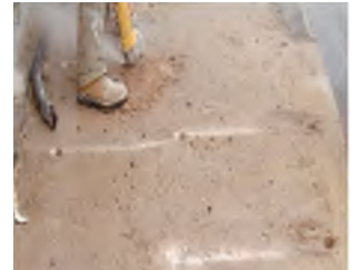
4 Interconnecting saw between anode holes and rebar connection location
