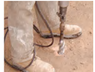
2 Drill holes for anode
