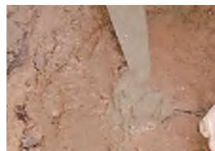
9 Cover top of anode and finish
