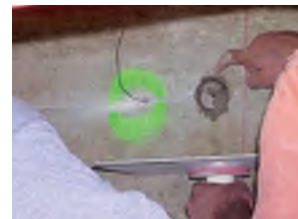
5 Press anode into mortar
