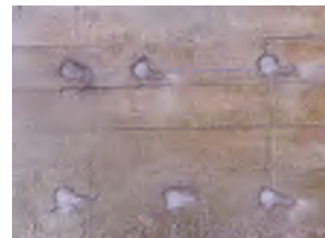
7 Top up mortar on anode and finish
