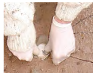
8 Install mortar and anode
