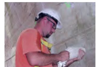
4 Place embedding mortar into anode hole
