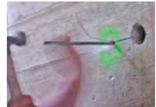
2 Install vector rebar connectors
