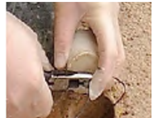
6 Connect anode to header wire
