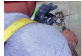
6 Connect anode and rebar connector
