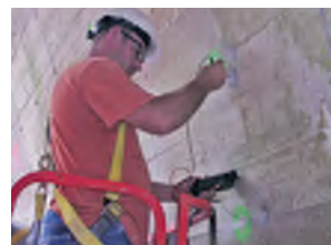
3 Verify rebar continuity between rebar connectors
