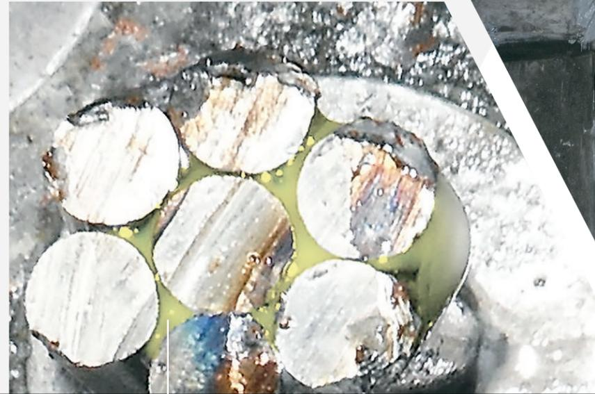
Example of impregnation being completed from the end of the tendon and the Post-Tech® PTI Impregnation material (highlighted in yellow) exiting the opposite end of strands 250 ft (75m) away.
