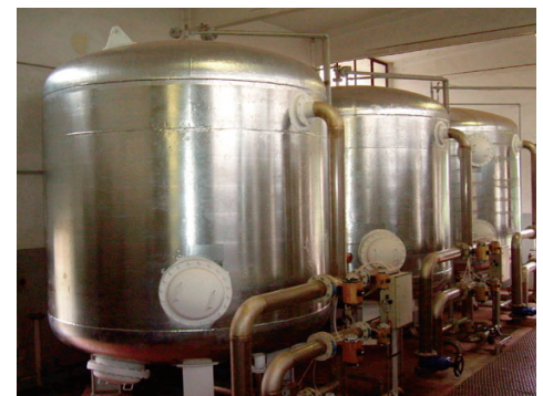
Condition of Tanks after ZincTape Application
