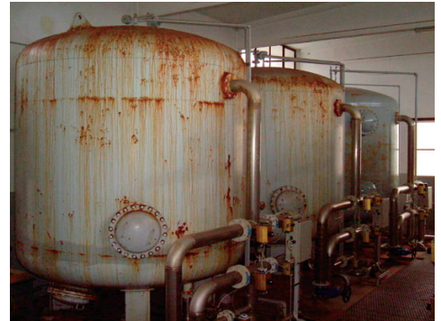
Condition of Tanks before ZincTape Application
