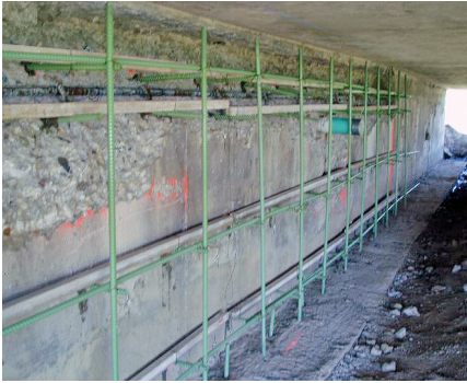
Galvashield® DAS Type C distributed anode system on corroded abutment prior to encasement with new concrete.
