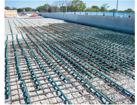
Galvashield® DAS distributed anode system on bridge deck prior to placement of reinforced concrete overlay.
