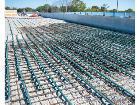
Galvashield® DAS Type F distributed anode system on bridge deck prior to placement of reinforced concrete overlay.
