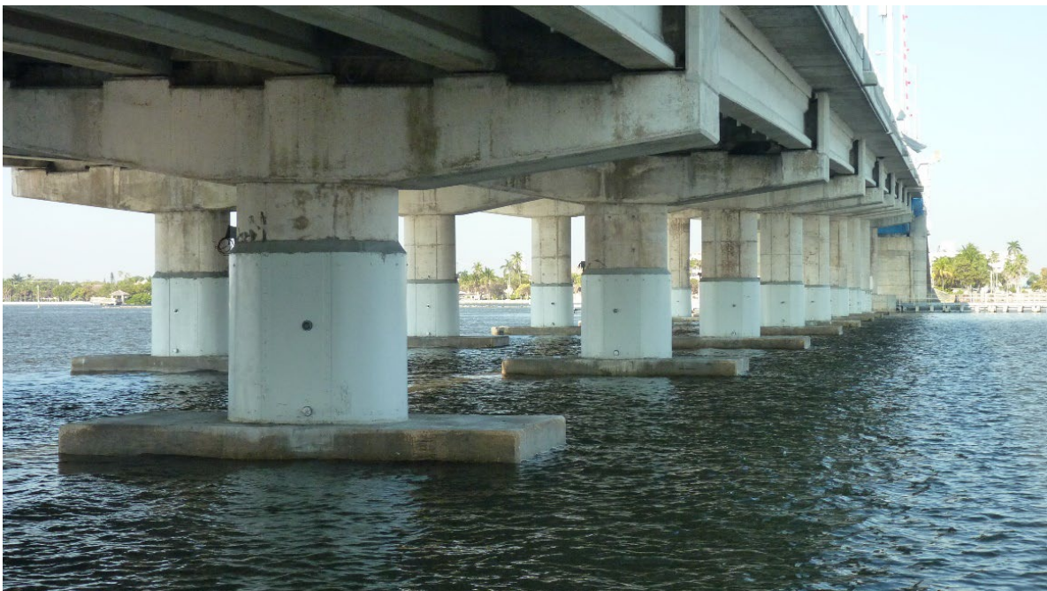
Figure 11: New Cathodic Protection Jackets Installed
