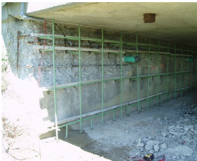
Figure 6: Galvanic Encasement of Abutment, Sidney, OH
