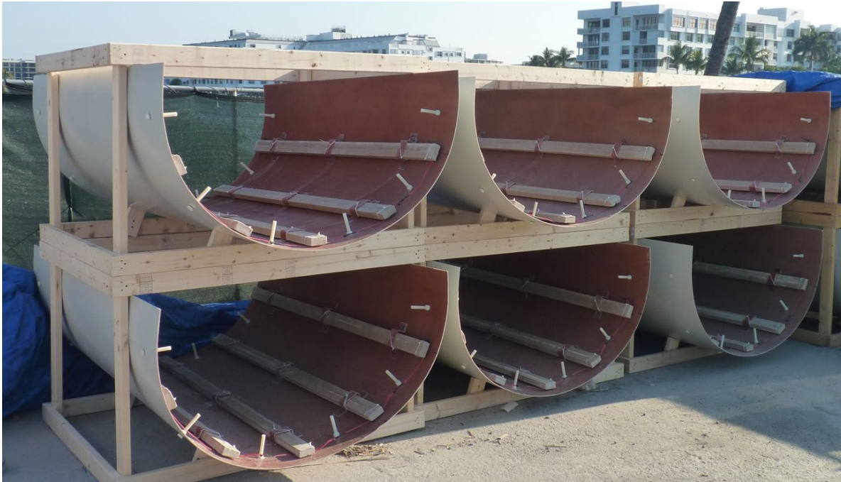
Figure 10: Curved Jacket Sections with Pre-Attached Distributed Anodes
