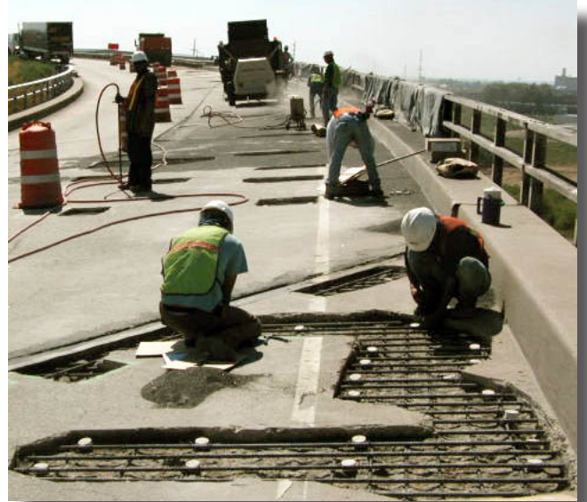
Installing Galvashield XP in bridge deck repairs
