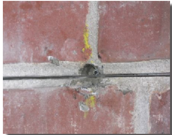
Ebonex anode installation
