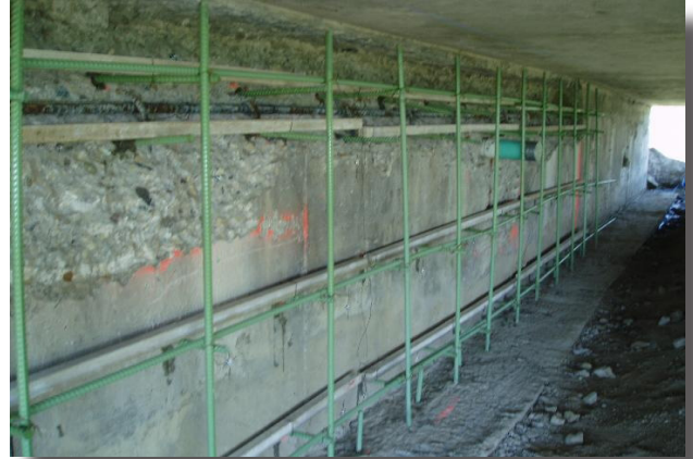
Galvanic anode system on bridge abutment prior to encasement in reinforced concrete overlay
