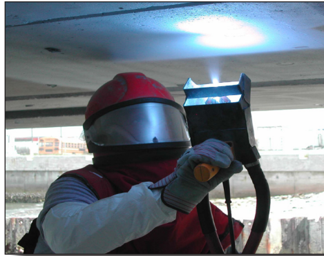
Galvanode ASZ+ on Precast Deck Units
