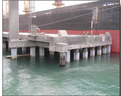
Galvanode Jacket for Pile Protection
