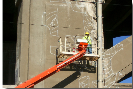
Delamination survey
