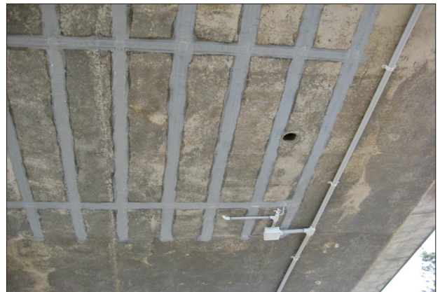
Ti Tape Anode Secured and Protected with FRP Tape
