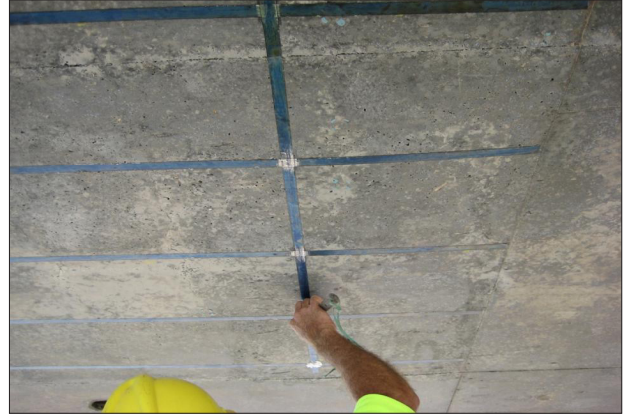
Mixed Metal Oxide Titanium Tape Anodes
