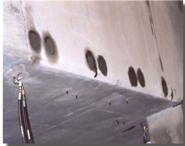
Post-Tech PT Grease Injection
