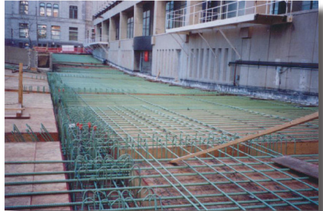
Galvashield installed at interface of new and existing concrete
