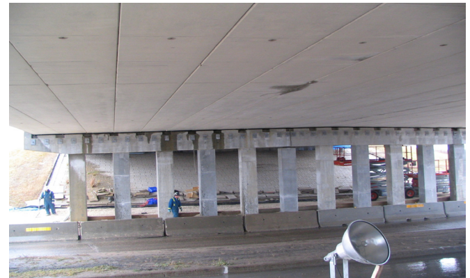
Pier caps jacketed with embedded Galvanode DAS anodes for corrosion control of chloride contaminated concrete
