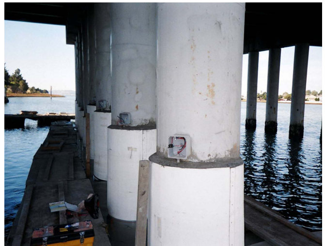
Galvanode DAS Marine Anodes inside stay-in-place FRP Forms
