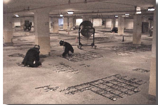
Anode units should be placed around the perimeter of the patch. (See data sheet for spacing guidelines)
