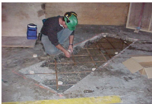
Anode units installed and ready for repair.
