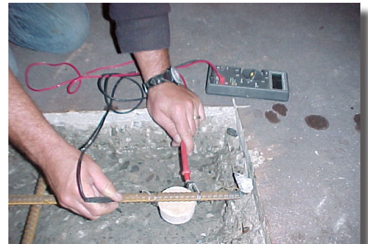
Check connection with a multimeter. Resistance should be 1 ohm or less.
