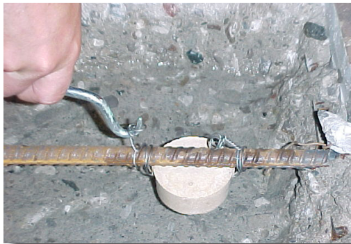
Tie the anode unit on the side or beneath the rebar providing minimum 3/4 in. cover and clearance on all sides
