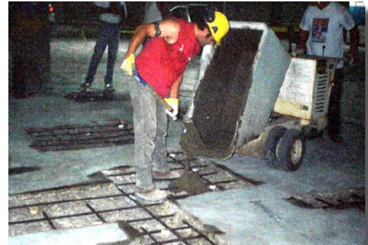
Complete the repair with compatible repair material.
