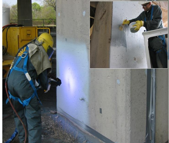
Photo of Galvanode ASZ+ installation and Galvanode humectant application (inset photo)
