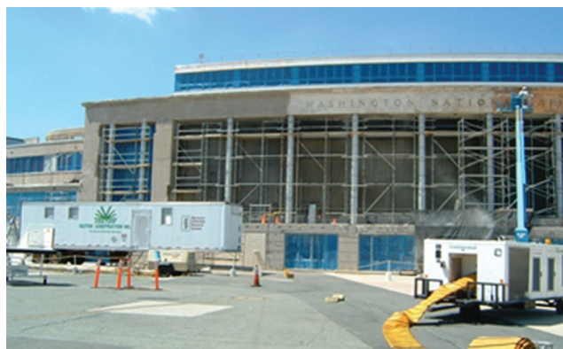
Fig. 4: Installation of realkalization system
