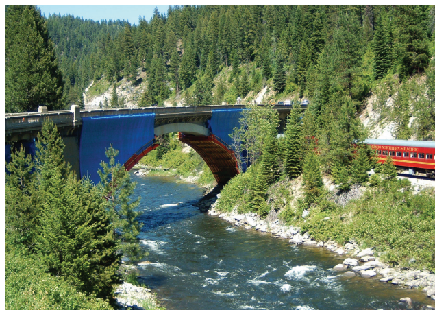
Fig. 6: Rainbow Bridge during rehabilitation
