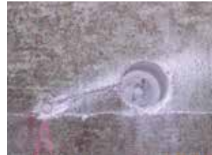
1 Saw cut between anode and rebar connection holes
