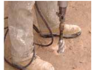
2 Drill holes for anode
