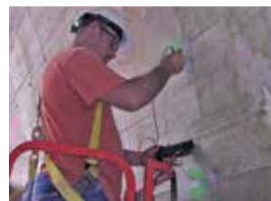
3 Verify rebar continuity between rebar connectors
