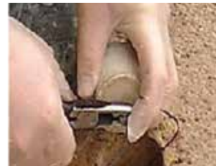
6 Connect anode to header wire
