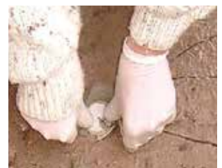
8 Install mortar and anode
