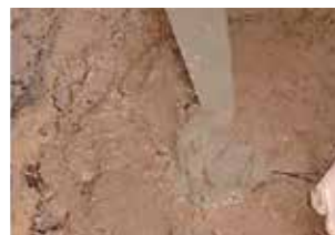
9 Cover top of anode and finish
