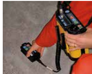
1 Locate steel and position anode
