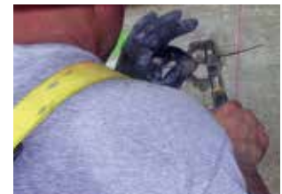
6 Connect anode and rebar connector
