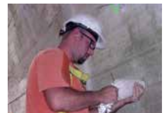
4 Place embedding mortar into anode hole
