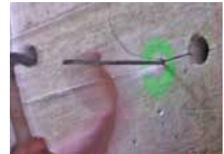
2 Install vector rebar connectors
