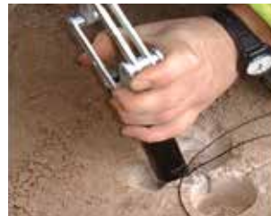
5 Pop rivet installation to steel
