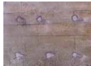
7 Top up mortar on anode and finish
