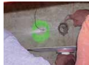
5 Press anode into mortar
