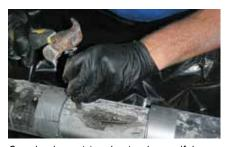
Opening in post-tension tendon verifying presence of Post-Tech PTI material around the strands
