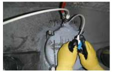
Post-Tech PTI impregnation occuring through the end cap of a post-tension tendon
