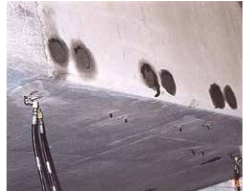
Post-Tech PT Grease Injection
