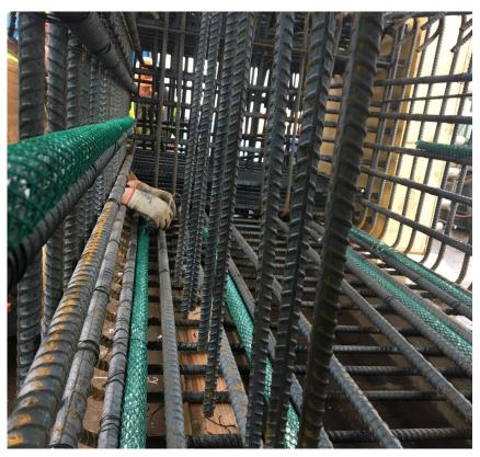
Galvashield® DAS installed into a new concrete beam prior to forming and casting.
